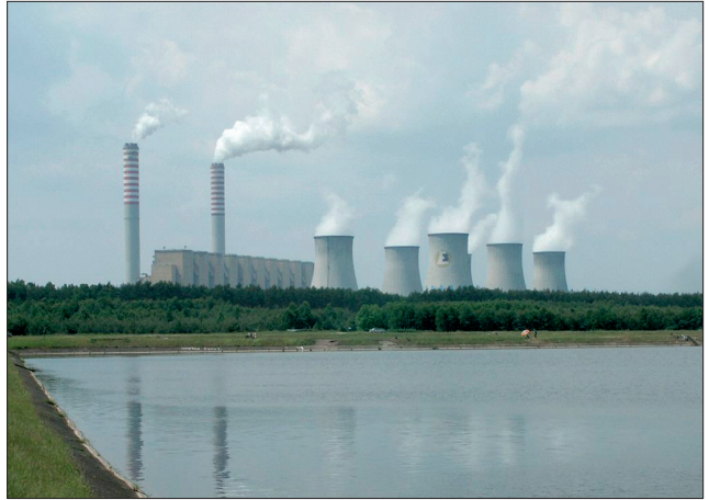
Figure 3.14. A coal power plant in Poland. Most of the visible emissions are just water vapor, but invisible gases include sulfur dioxide ( \text{SO}_2 ) and various nitrogen oxides. Combustion of coal also produces a tremendous amount of carbon dioxide, a greenhouse gas.
